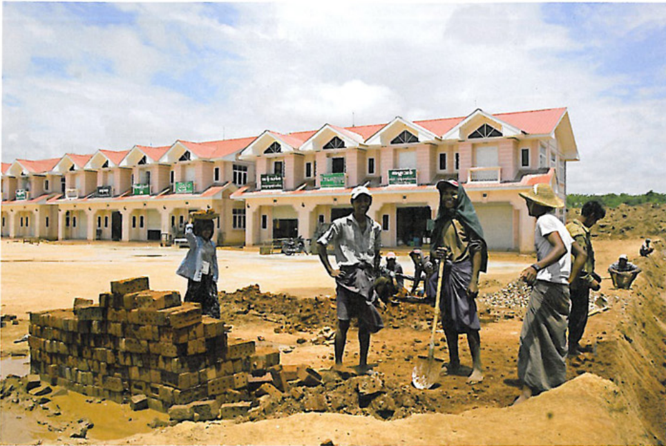
Ill-equipped workers dig a ditch beside new storefronts.
